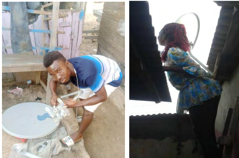
Figure 12 Beneficiaries learning to install a TV signal receiver
