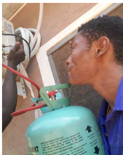
Figure 13 Trainee on installation of an air conditioner
