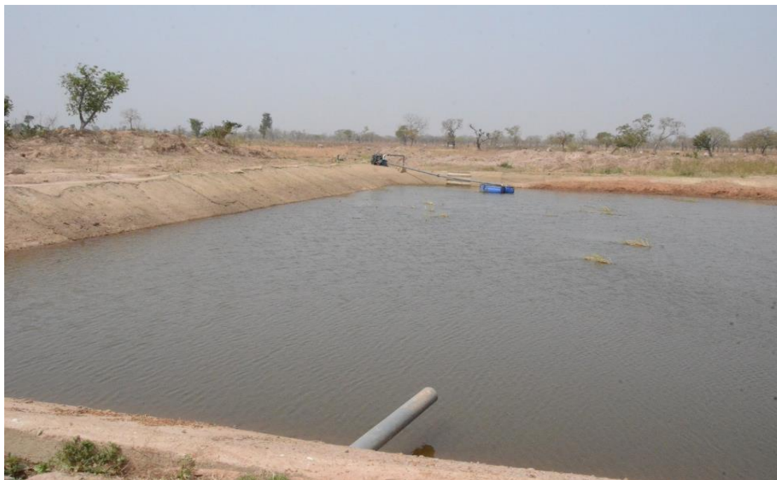
Wambong Dam Irrigation Facility after rehabilitation
