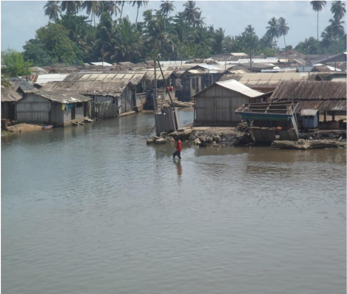
Figure 6 Buildings close to the Ankobra River in Sanwoma community
