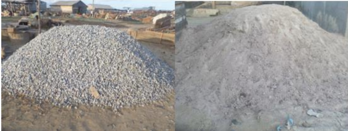
Figure 4: Some materials used in securing the footing of the racks during the construction process
