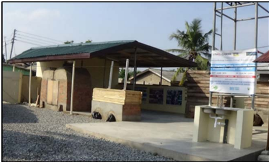
Figure 8 Refurbished Interim DFTC (DAA Fisheries Training Center)
