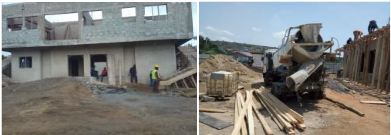
Figure 20: DAA Fisheries Training Center under Construction
