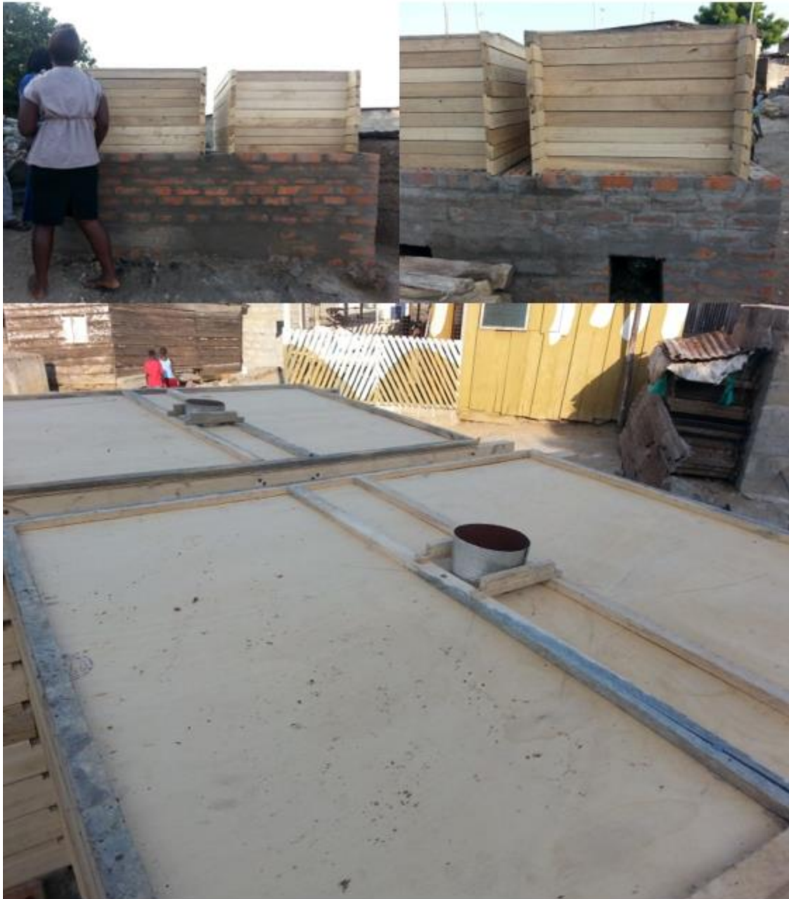
Figure 2. A finished constructed Morison Oven for fish processors in Winneba in the Central Region of Ghana.
