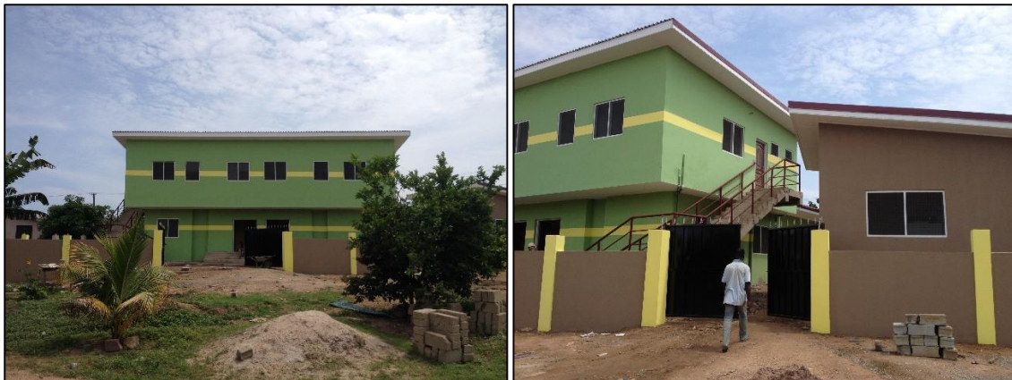
Figure 5. Pictures of the almost complete DAA Fisheries Training Center building
