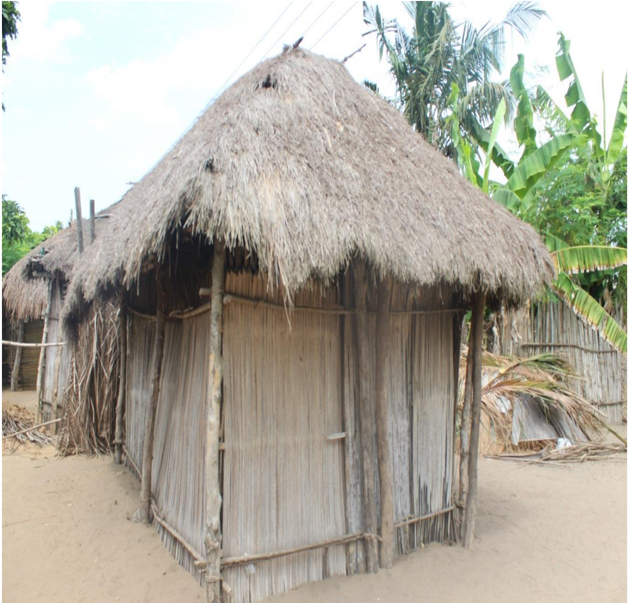
Figure 8 A structure built with bamboos and mangrove trees
