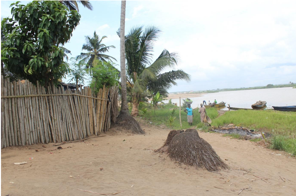
Figure 4 showing structure which is very close to river Pra and exposed to flooding
