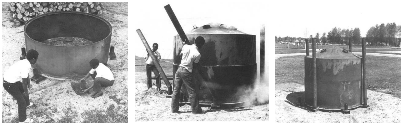
Figure 7. Metal mobile kiln under assembly
