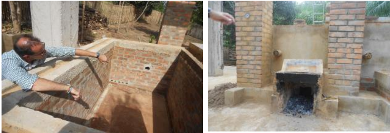
Figure 6. Interior view (left) and front view (right) of the concrete/brick kiln
