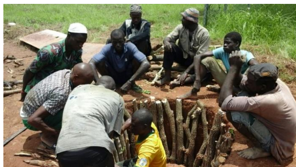
Photo 27 Lining of latrine pits using local materials (Karaga District)
