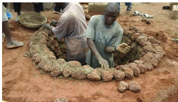
Photo 28 Lining of latrine pits using local materials (Karaga District)
