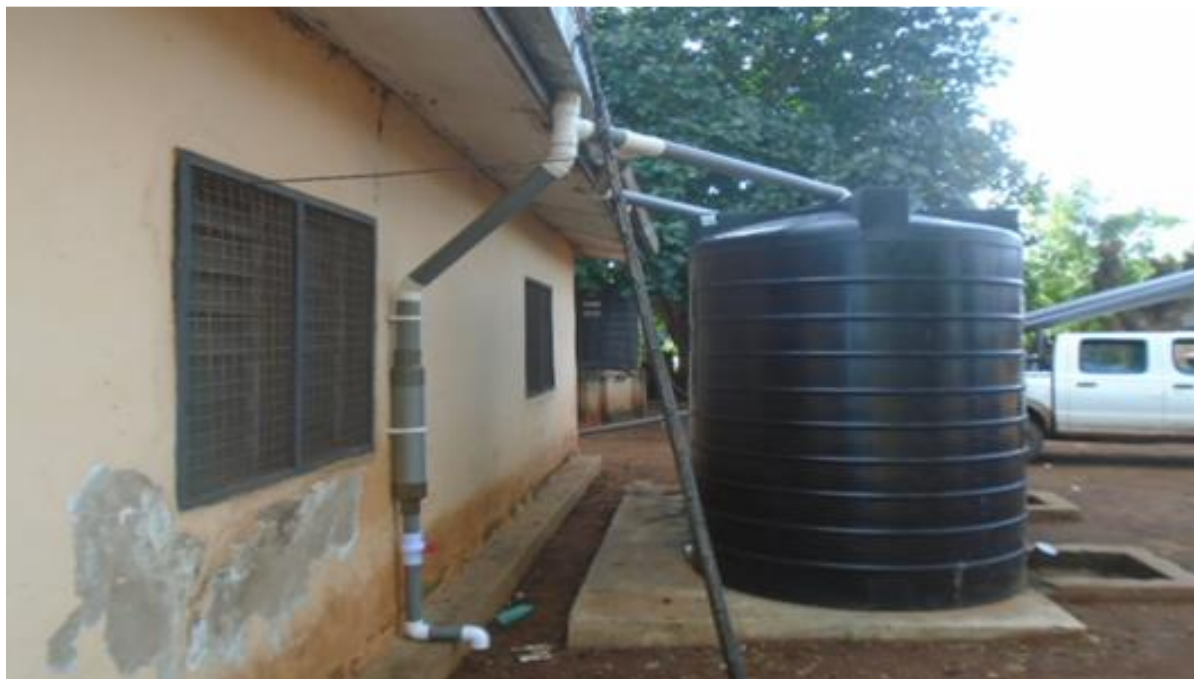
Photo 31 Installed systems with 4,000L holding capacity at Wantugu Health Centre in Tolon District
