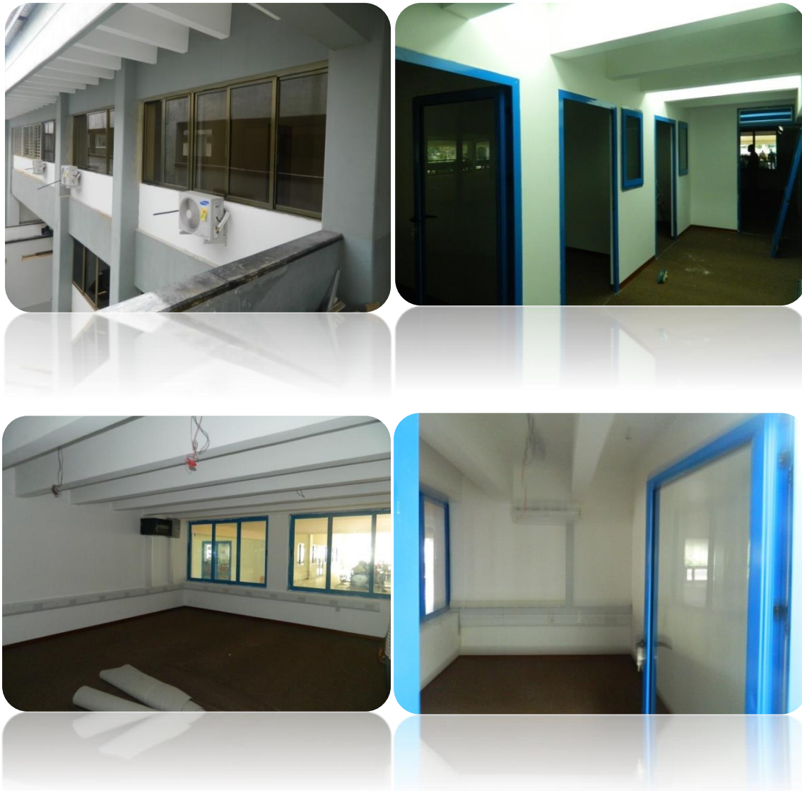
Figure 17: Refurbished Spaces Designated for the Centre for Coastal Management (CCM)
