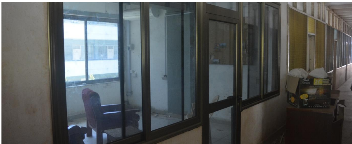
Figure 9: Offices being refurbished for DFAS lecturers to enhance teaching and learning
