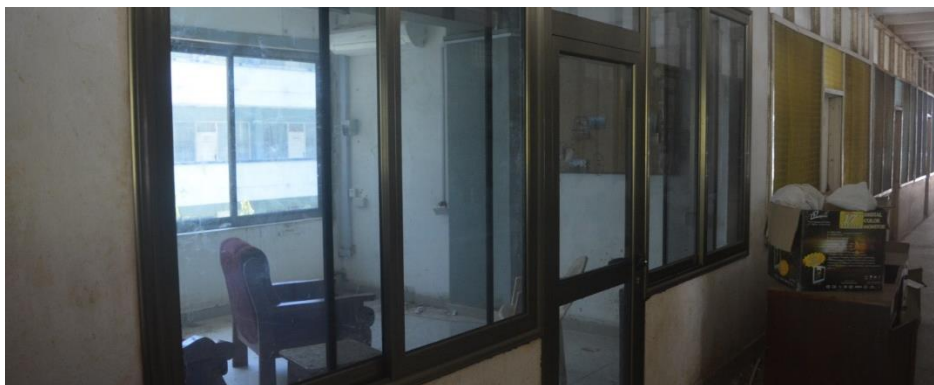
Figure 14: Offices being refurbished for DFAS lecturers to enhance teaching and learning
